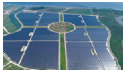
Solaseado Solar Power Plant
