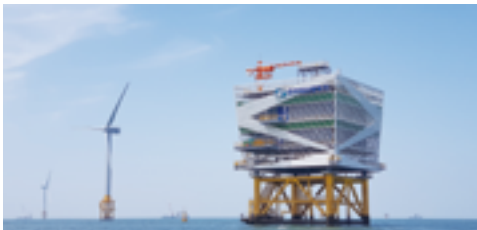
Southwest Sea Offshore Substation
